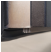
lip seal, rebate with seal
